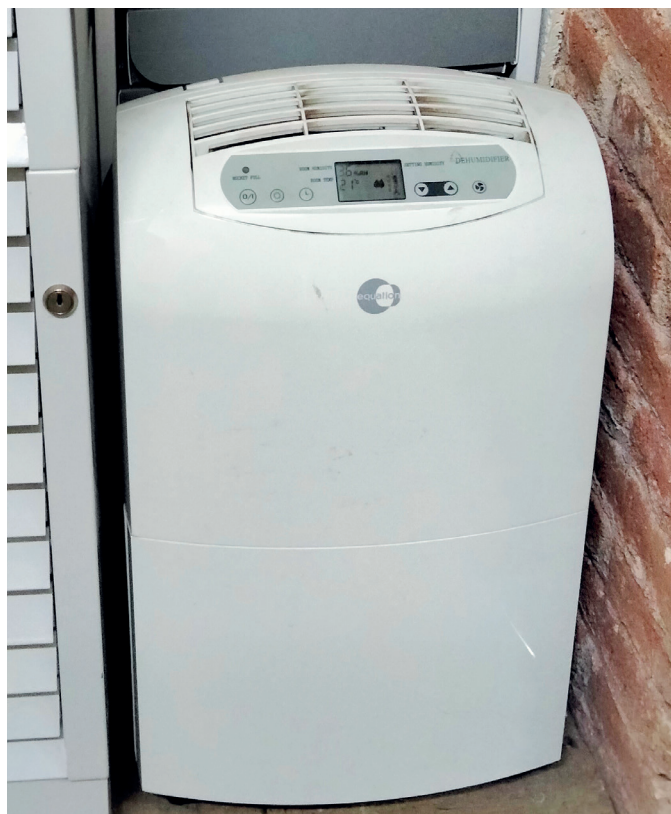
Figure 16. When economical resources are scarce, nowadays there are cheaper options that could help to control at least maximum and minimum temperature and humidity, which are the most critical variables to monitor. Source: Observatori Fabra.
