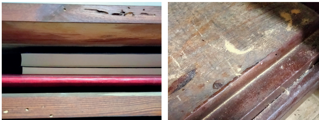
Figure 18. Cleaning with a known periodicity also helps to detect possible infestations or other problems and determine since when they could exist or not.
